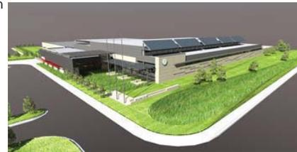
A rendering of the Quad Cities MetroLINK Transit Maintenance Facility displays the solar panels, bio-swale and high-efficiency roof, which administrators hope will make the structure a beacon for green design in the area.
